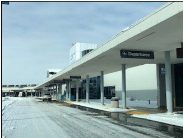
SBN terminal building curbside
