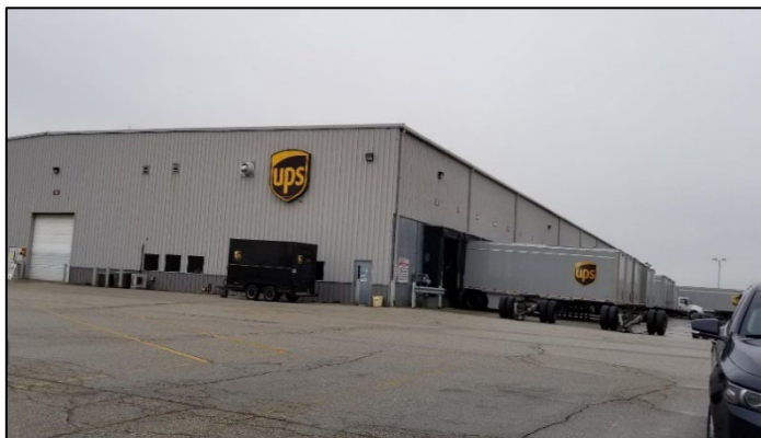
UPS facility at SBN
