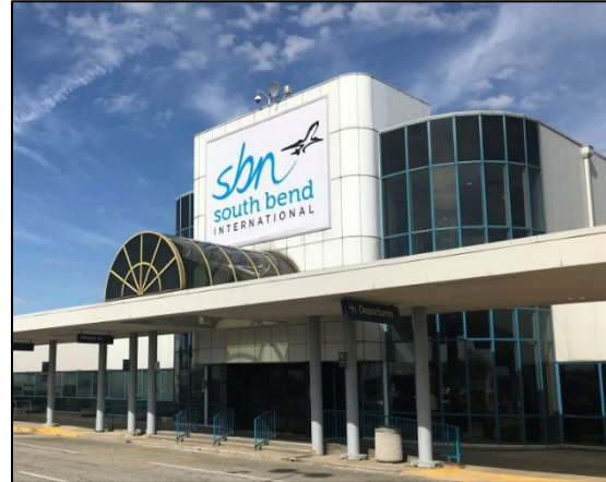
SBN terminal building Source: Northwest Indiana Business Magazine
