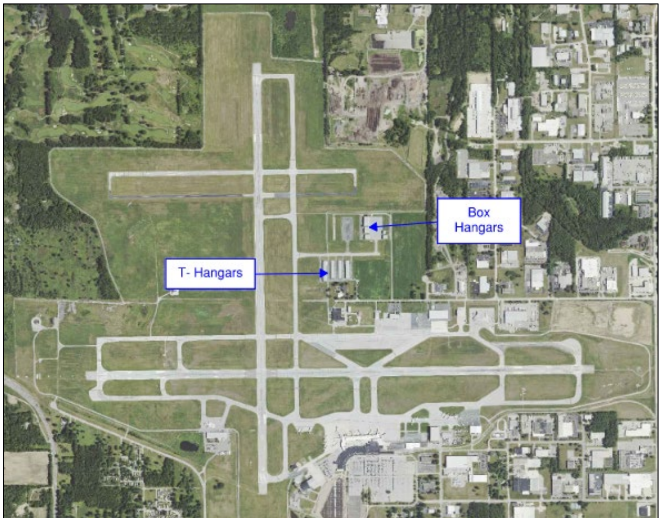
Figure 1-14: Aircraft Hangar Locations
