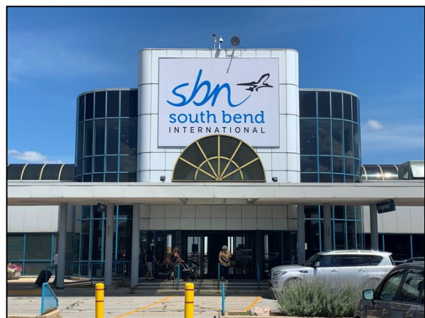
SBN terminal building
