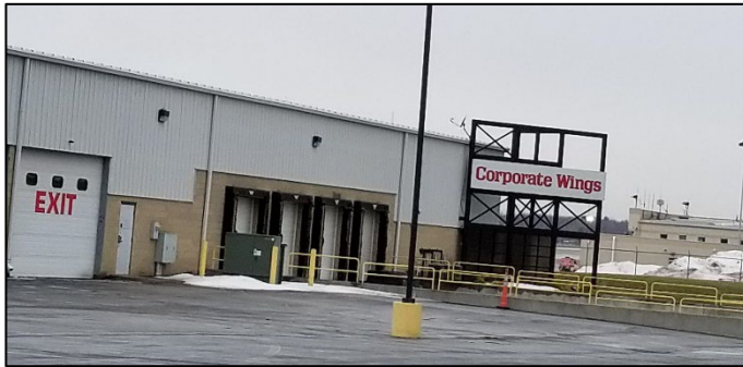
Corporate Wings facility at SBN
